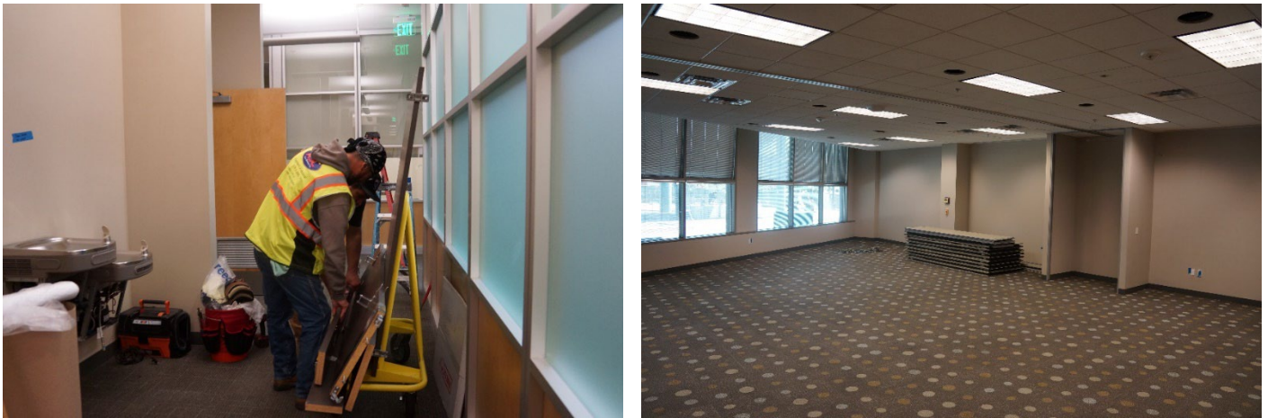
Commencement of Office-Space Conversion into Shelter October 8, 2024
