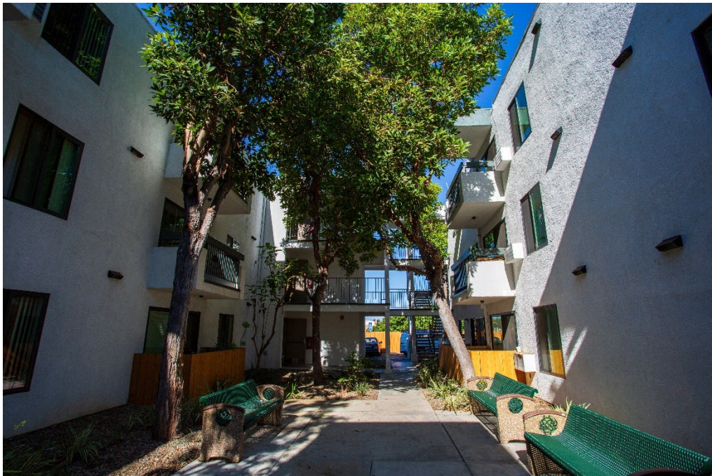
Park Crest Senior Apartments SDHC-owned Affordable Rental Housing
