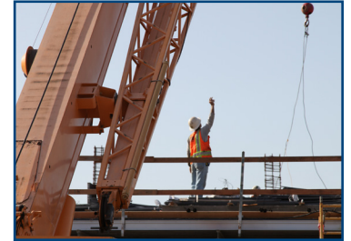
Construction work on affordable housing
