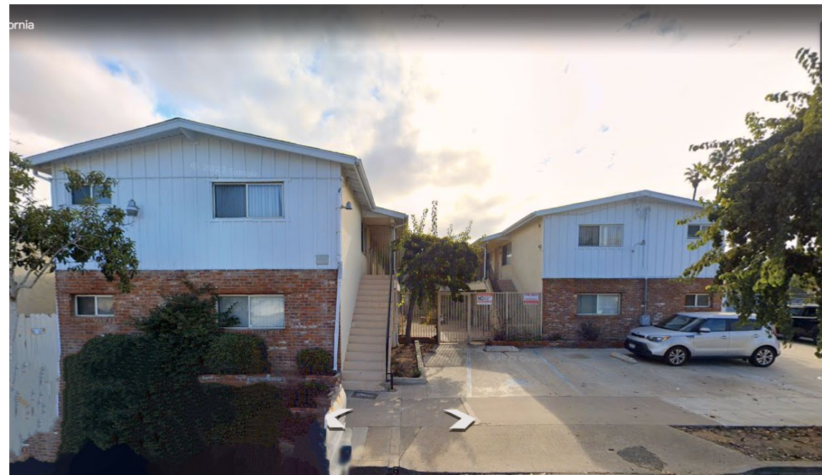
Street view of 2147 Abbott Street
