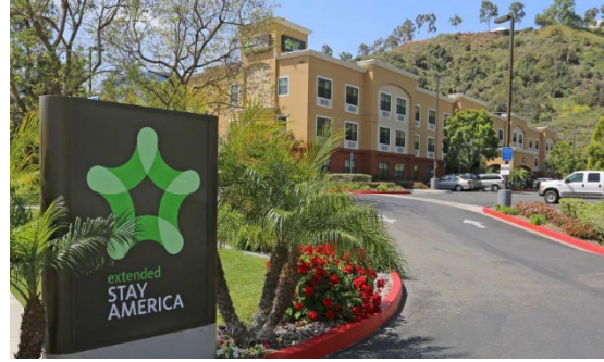
3860 Murphy Canyon Road Council District 7
