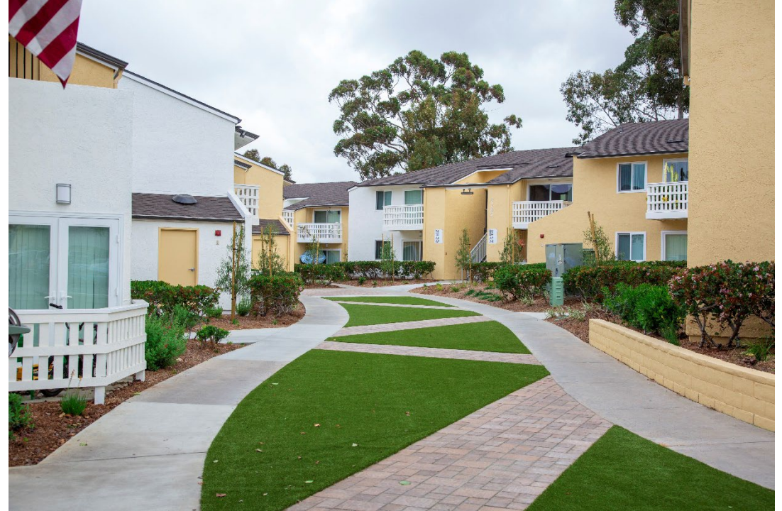
Village North Senior Garden Apartments SDHC-owned affordable housing Council District 6
