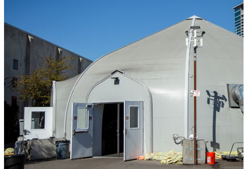
City of San Diego Bridge Shelter 1501 Newton Avenue February 22, 2019
