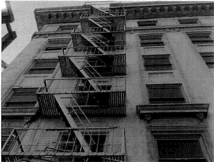
Exterior elevation showing fire escape.
