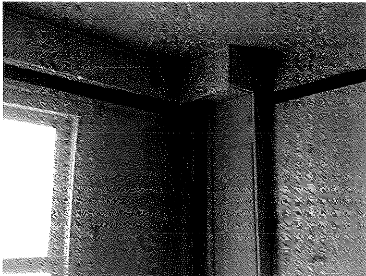
Unit drywalled soffit and chase for electrical rough additions.
