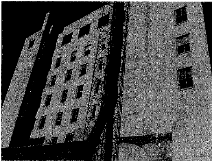
Exterior elevation of rear building showing trash chute.
