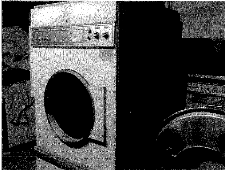
Existing commercial laundry dryer in basement.
