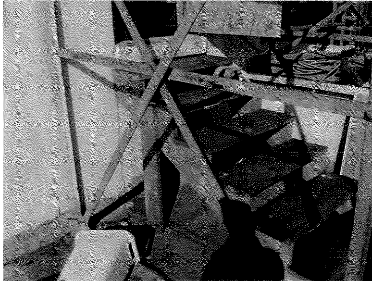
Steps to elevator machine room.
