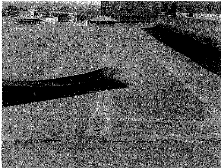
Existing flat roof (to be replaced)
