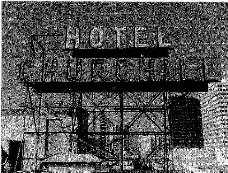
Rooftop sign (to be refurbished)
