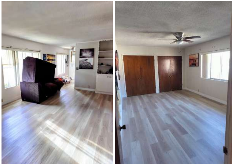
[PHOTO: Vinyl flooring installation showing complete removal of carpet]
