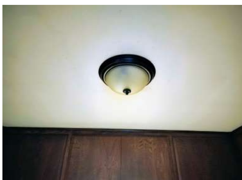
[PHOTO: Kitchen ceiling fixture installed by Townspeople]
