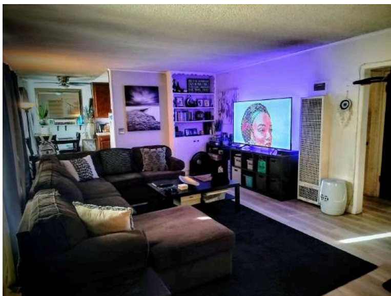
[PHOTO: Taken after vinyl installation showing dark soot contamination across ceiling, July 16, 2024]
