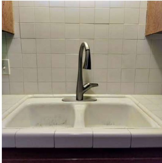
[PHOTO: Full view of kitchen sink showing degraded dual basin with modern replacement faucet installed over deteriorated fixture, Feb 14, 2026]
