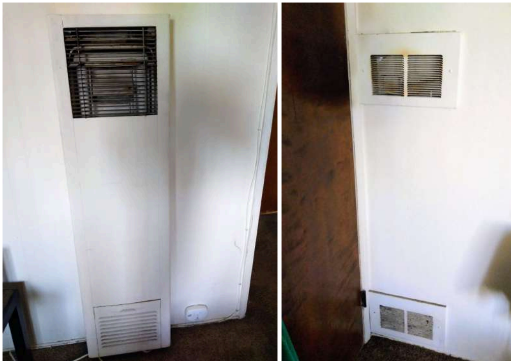
[PHOTOS: Original furnace showing BOTH vents - upper living room and bedroom, bedroom door visible soot contamination Dec 15, 2019]
