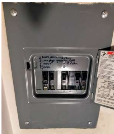
[PHOTO: Circuit breaker box replaced under [REDACTED]]
