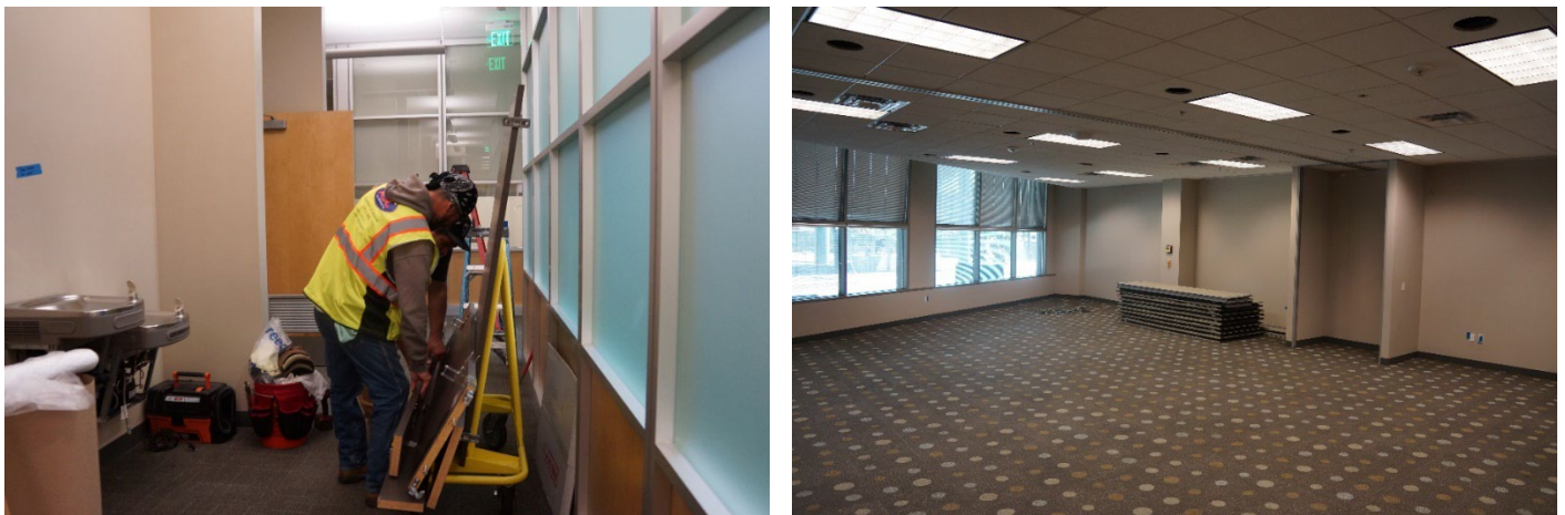
Commencement of Office-Space Conversion into Shelter October 8, 2024
