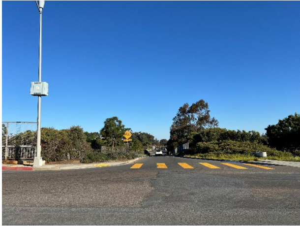
View of Nimitz Boulevard on ramp facing northwest
