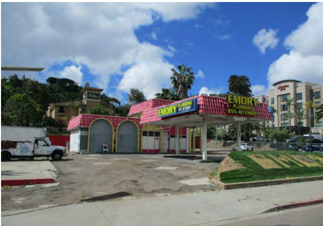
Properties adjacent to west of Subject
