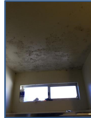
Moisture on ceiling from water leak
