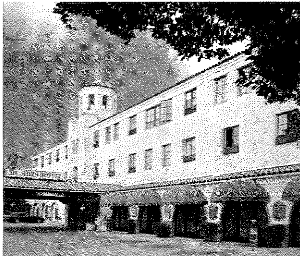
De Anza Hotel, an urban restoration project.
