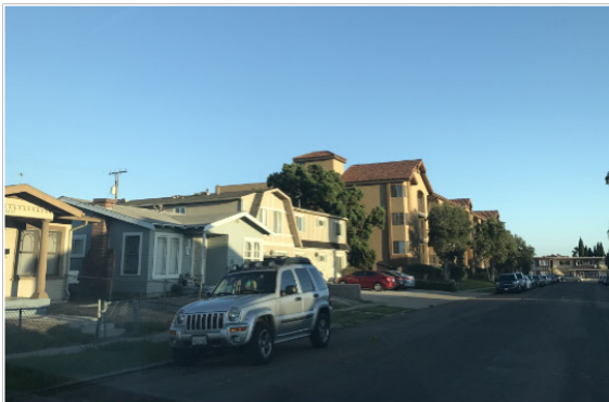
Existing dense, multifamily construction alongside single-family homes by El Cajon and 35 th Street
