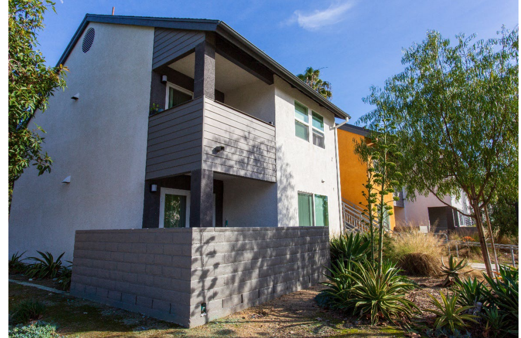
SDHC Affordable Housing Property – Via Las Cumbres
