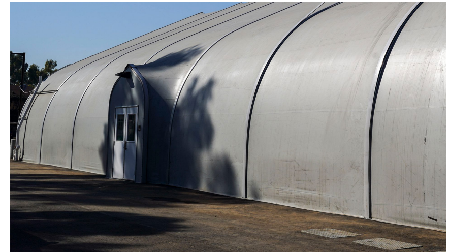
Imperial Shelter for Single Adults Exterior of the Imperial Shelter for Single Adults at 1710 Imperial Avenue, San Diego, CA 92101
