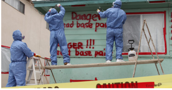
A 1941 Linda Vista home receives lead-based paint remediation.
