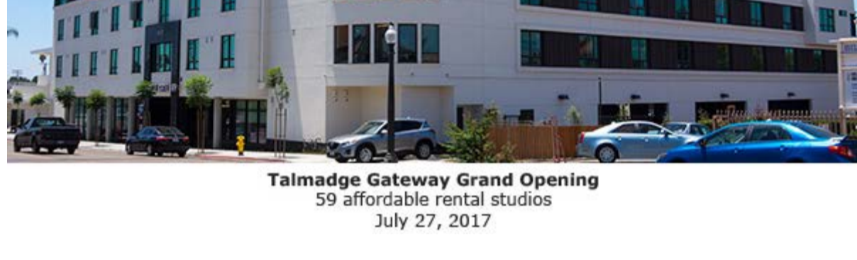
Talmadge Gateway Grand Opening 59 affordable rental studios July 27, 2017
