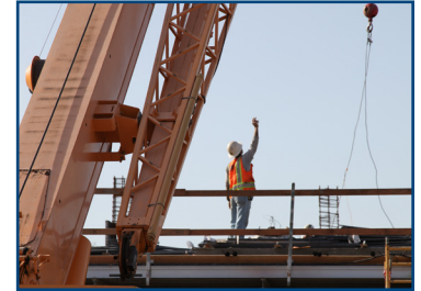
Construction work on affordable housing
