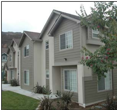
SDHC’s Golfcrest Drive site is a former public housing property that the agency transitioned to a voucher-based program.
