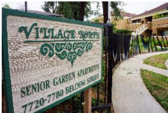
Village North Senior Garden Apartments 120 units – 44 units for homeless seniors HOUSING FIRST – SAN DIEGO
